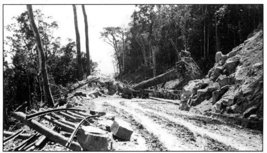
partly concealed behind ca1933 Mt Spec Road. View of a large maple balanced on the edge of Mt Spec Road during construction. Note the some rocks and bushes, use of mining technology – tramlines and trolleys.
