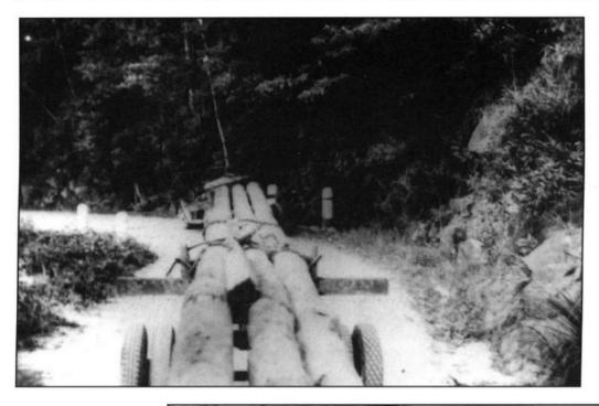
1943 Mt Spec Road. 100 foot White Gum. Logs for wartime radio masts had to be lifted around the many corners of the Mt Spec Road. Once at the bottom of the range the logs were loaded onto railway wagons at either Moongobulla or Rollingstone Stations.
