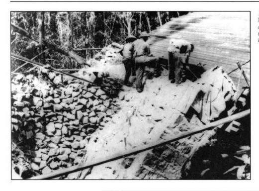
10 October 1932 Little Crystal Creek, Mt Spec Road. Abutment 'B' looking due south. Note the lagging put down on the formwork to hold the concrete when it was poured over the rock fill.
