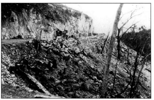
Blasting powder was used to ca 1933 Mt Spec Road at 45,000 feet through chainage. Stone cutting during construction. Mrs McClelland noted that it was their car.
