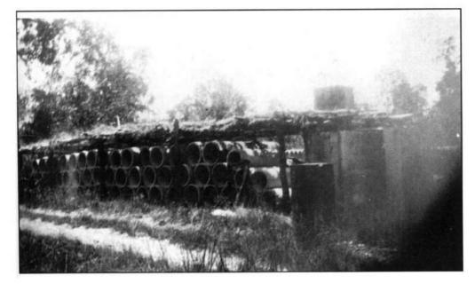
1932 Ollera Creek Pipeworks, Mt Spec Road. Pipeworks curing shed with stored pipes. Note the bough shelter over the curing concrete pipes. If the concrete dried too quickly, its strength was effected. McClelland, Thuringowa Collection
