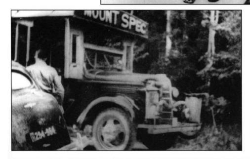
ca 1942 Paluma. Mt Spec bus with gas generator fitted. Petrol supplies were strictly rationed during the war.
