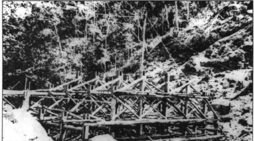
Early 1932 Little Crystal Creek, Mt Spec Road. Note the use of the round timbers for the initial framework of the masonry arch bridge.
