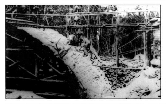
10 October 1932 Little Crystal Creek, Mt Spec Road. Abutment 'B' looking due South. Note the rock fill behind the arch.
