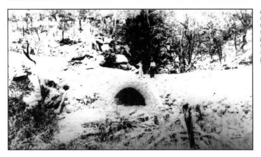
ca 1932 Mt Spec Road. A smaller masonry arch culvert at 17,100 feet through chainage. Through chainage was measured from the beginning of the project at Moongabulla (near today's turnoff at Ollera Creek). There are several stone culverts like this. This particular one is at the base of the range. This was Job Number 117-501-4.
