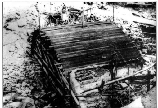
10 October 1932 Little Crystal Creek, Mt Spec Road. Construction of the masonry arch bridge. Abutment 'B' in the foreground. Note the use of sawn hardwood for the final formwork. Work was delayed while stocks of sawn timber were delivered on site.
