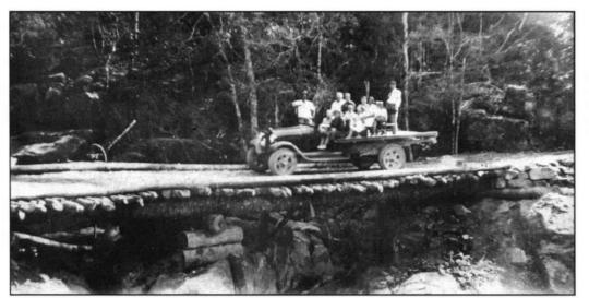
ca 1933 Little Saltwater (Crystal) Creek, Mt Spec Road. Ford truck on temporary bridge over Crystal Creek. This timber bridge was erected to provide access to works beyond Little Crystal Creek while the masonry arch bridge was still under construction.
